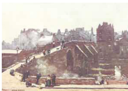
Figure 4: Auld Brig of Ayr; note cutwaters and narrowing of roadway.
